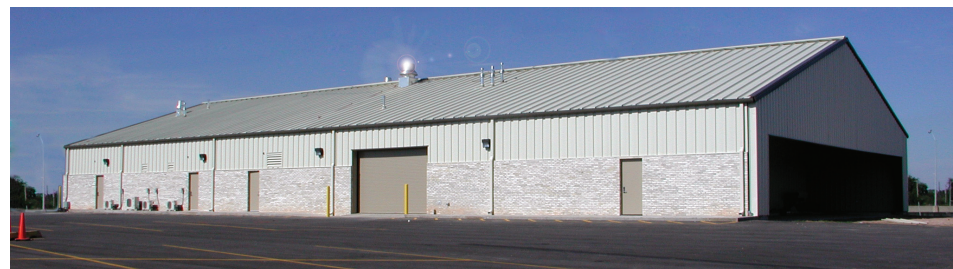
OSU-OKC Physical Plant Building
